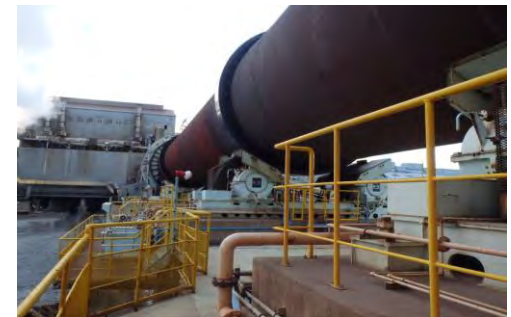
Rotary kiln in operation (at PAMCO)
